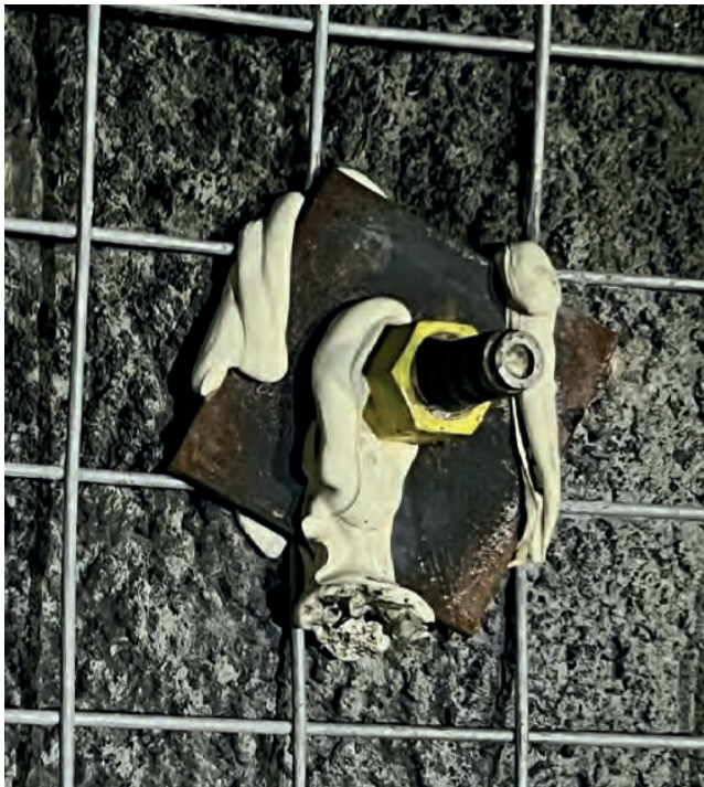
Figure 1. SDA bolt installed in highly fractured ground.
