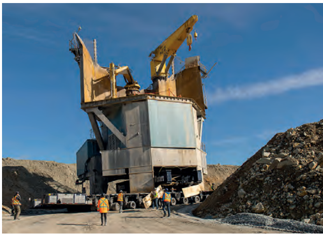
Figure 4. Relocation of a TAKRAF semi-mobile crushing station in Canada. Entry into the new pocket area.
