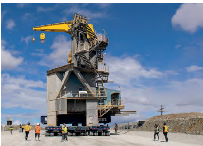
Figure 2. Relocation of a TAKRAF semi-mobile crushing station in Canada. This was also the first crushing station to be supplied by TAKRAF’s Canadian operation.
