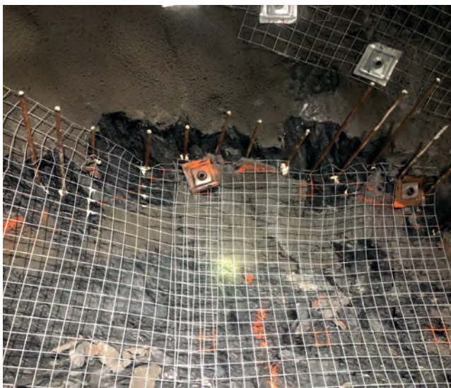
Figure 4. Spiling with PUS MasterRoc RBA.
