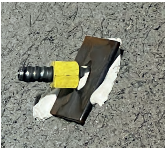
Figure 2. Installed bolt with MasterRoc RBA.
