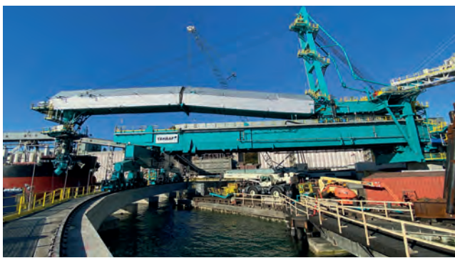
Figure 5. Quadrant beam ship loader in the park position on site at the Port of Vancouver.
